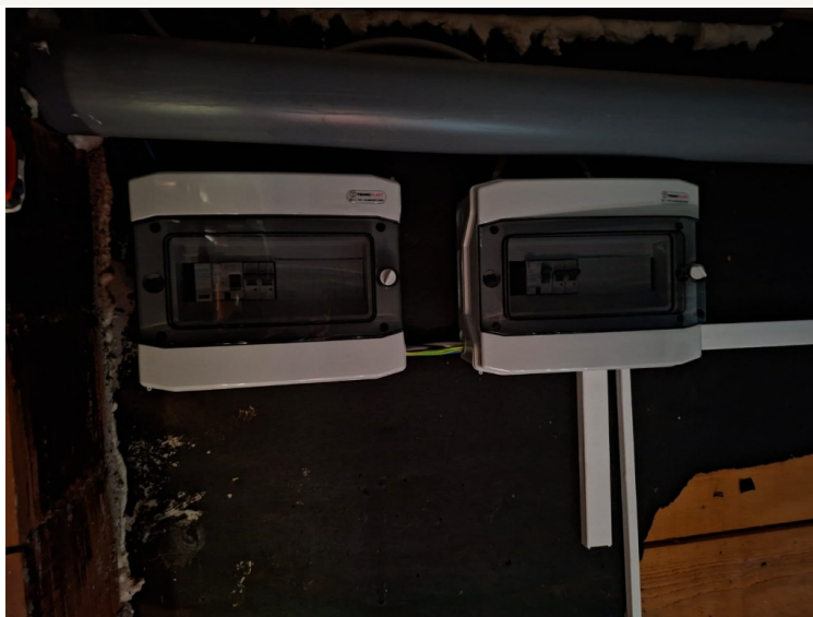
The left electrical cabinet in the boiler room.
